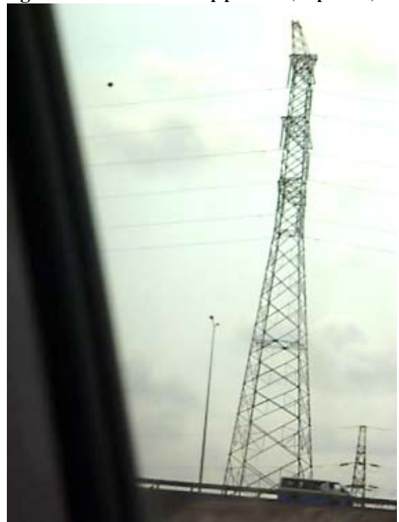
Figure 7-12 220 kV steel angle tower
