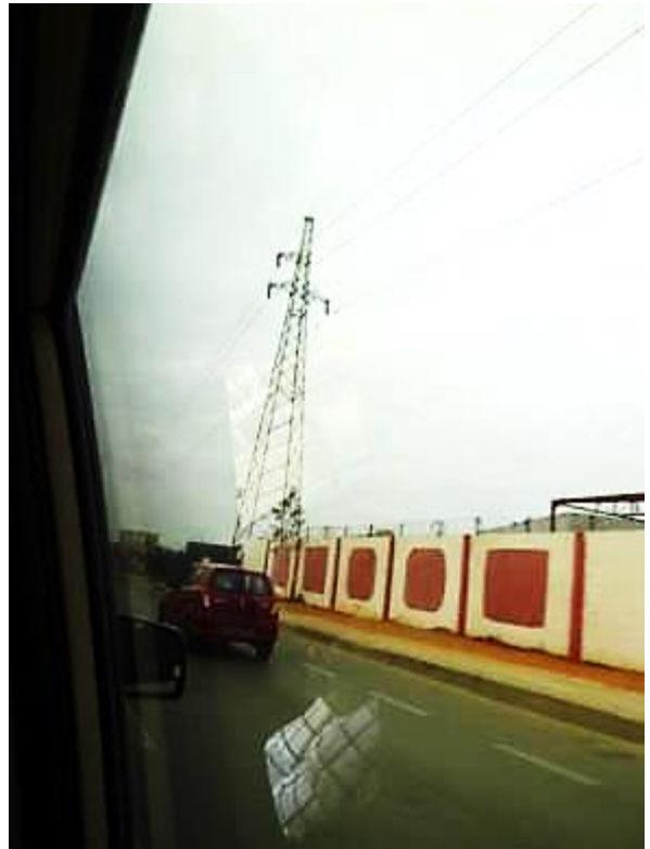
Figure 7-6 66 kV one circuit angle tower
