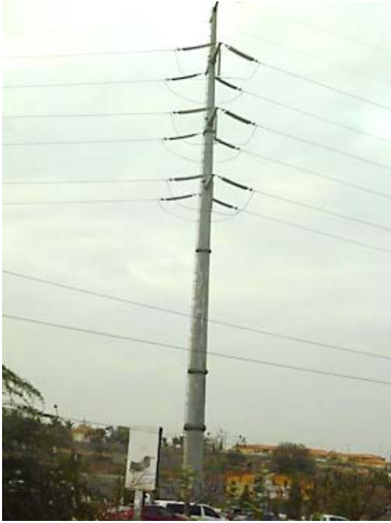
Figure 7-9 220 kV steel pipe tower (tension)
