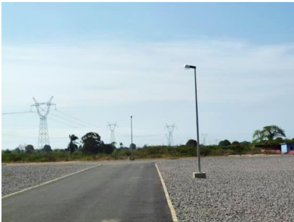
Figure 7-13 400 kV one circuit transmission lines (distant view)
