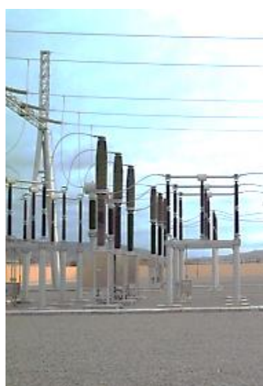
Figure 7-16 220 kV vertical type gas-insulated circuit breaker
