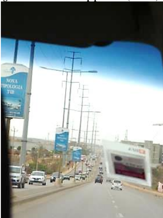
Figure 7-11 220 kV Transmission line along the road
