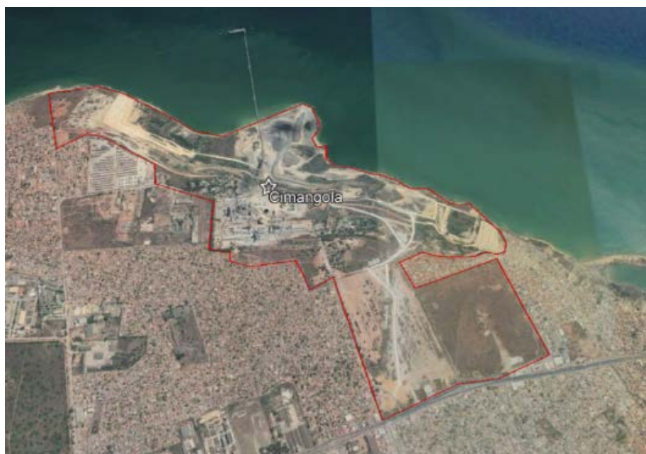
Figure 11-8 Site for CIMANGOLA Thermal Power Plant
